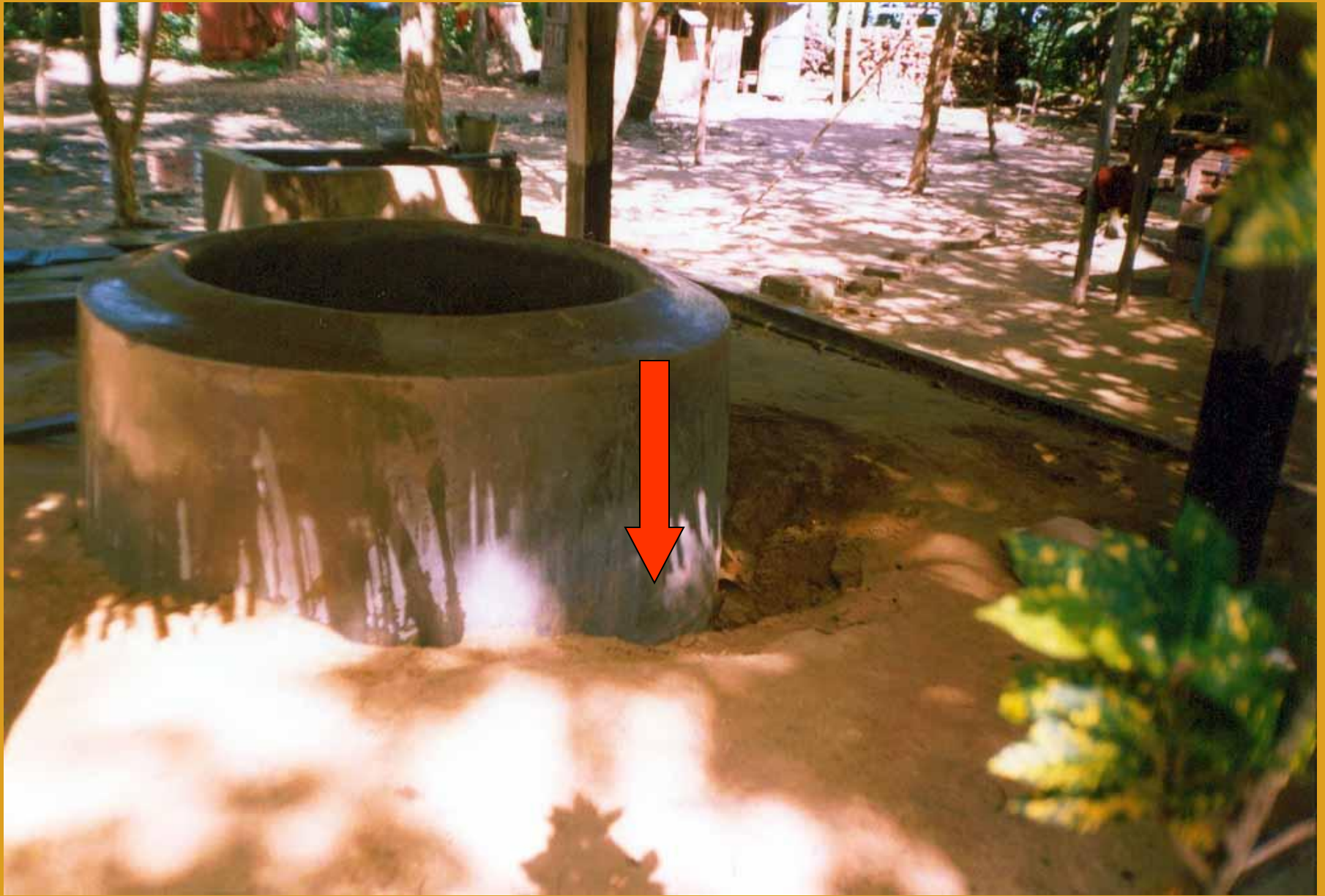
Evidence of Ground failure
